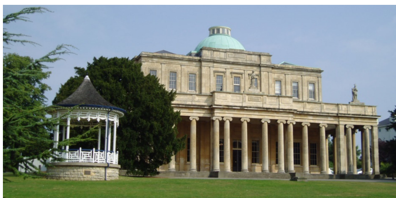
Pittville Pump Room
