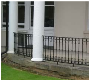
The colonnade at the rear of Hygeia House provides the earliest accurately dateable ironwork in the town
