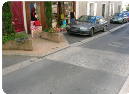
Build-out with courtesy crossing and planting
