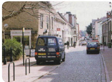
Surface treatment with build-out that defines parking bays.
