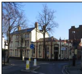
Figure 31 St James Hotel building
