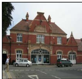
Figure 28 The Crescent Bakery building
