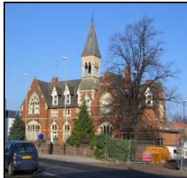
Figure 30 Dowty House building
