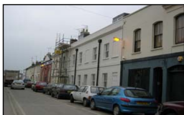
Figure 22 Terraces in Bennington Street
