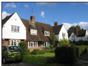
Figure 42 Shallow dormer windows on roof slopes of houses in Kingsley Gardens
