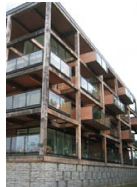
The Accordia development in Cambridge incorporates lower ground floor parking screened by granite gabions allowing light and ventilation
