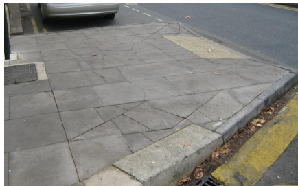
Damaged paving
