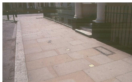
Paving laid perpendicular to the kerb
