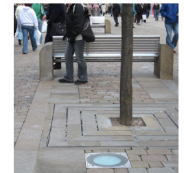
Tree surround with paving infill
