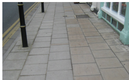
Avoid laying paving parallel with kerb which emphasises lines and the number of joints
