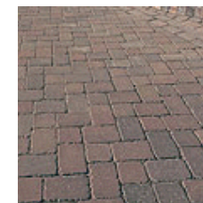
Tumbled concrete blocks
