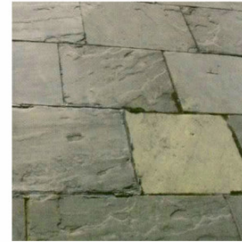
Natural Yorkstone paving 600mm wide x random length with riven finish
