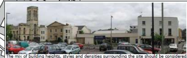
The mix of building heights, styles and densities surrounding the site should be considered.
