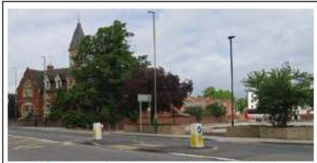
Threshold between Dowty House and the site needs to be addressed to respect residential amenity.
