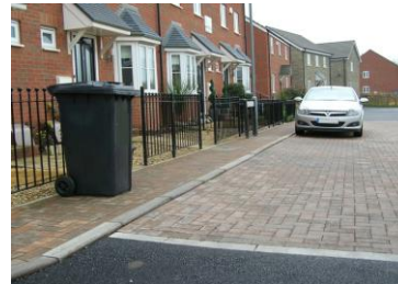
Pavers must be able to withstand the weight of collection vehicles; drop kerbs assist the movement of bins
