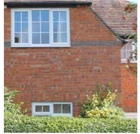
Fig.5.16 Horizontal tile creasing
