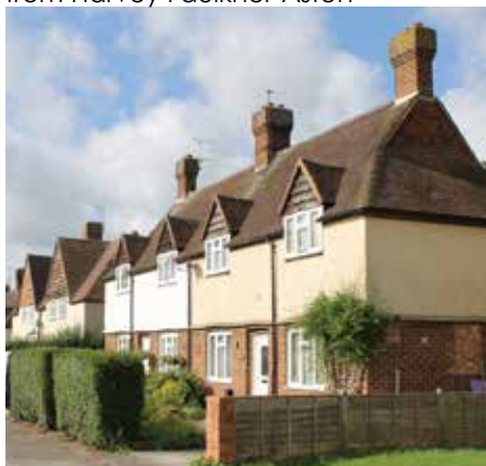
Fig.5.33 Stepped Chimneys Shelley Avenue
