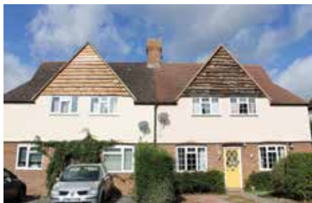
Fig.5.28 Horizontal boarding on gables
