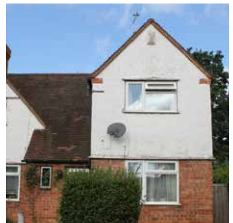
Fig.5.30 Catslide roof and brick detail- ing and string cornice
