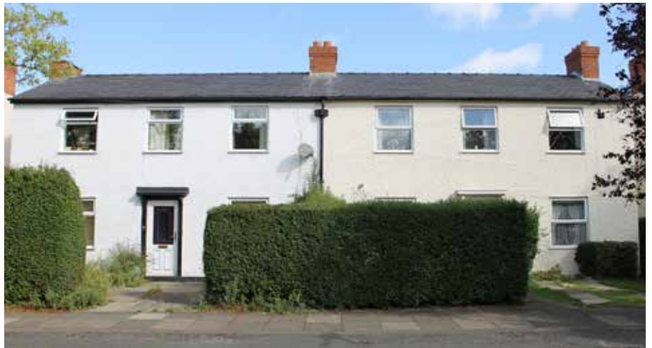
Fig.5.2 Dorlonco Houses with roughcast render, slate roofs and cast iron rainwater goods
