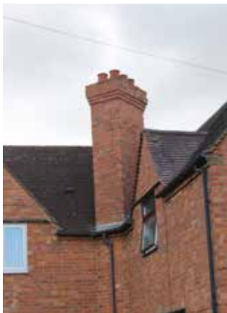
Fig.5.19 Tall stepped chimney
