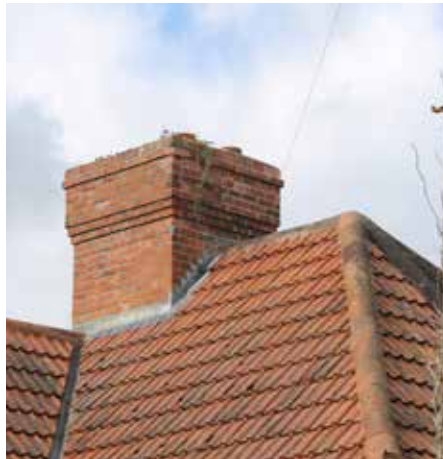
Fig.5.26 Centrally located chimney Spencer Road and Bridgewater tiles
