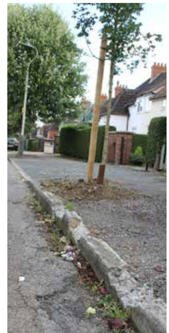
Fig.4.5 Poor condition of concrete kerbs
