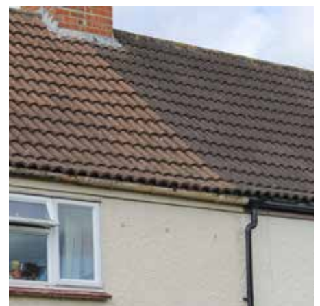
Fig.5.9 Original and replacement pantiles
