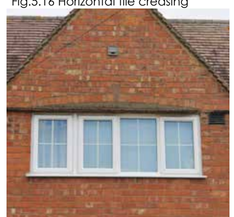
Fig.5.18 Plain gable with relieving arch over window
