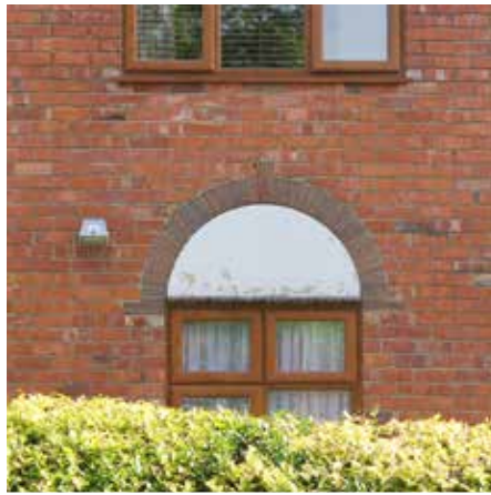
Fig.5.13 Rendered infill panels
