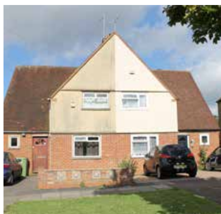
Fig.5.34 Catslide roof with flat clay tiles
