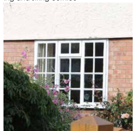
Fig.5.32 Original timber windows
