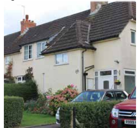
Fig.5.6 Forward projecting half storey
