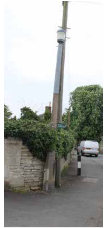
Fig.4.12 Street lighting and clutter
