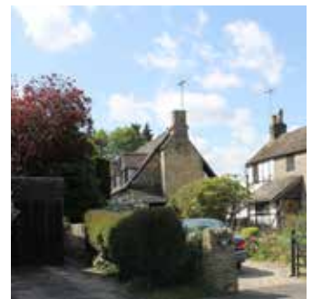
Fig.3.1 Houses following the original Burgage plot boundaries
