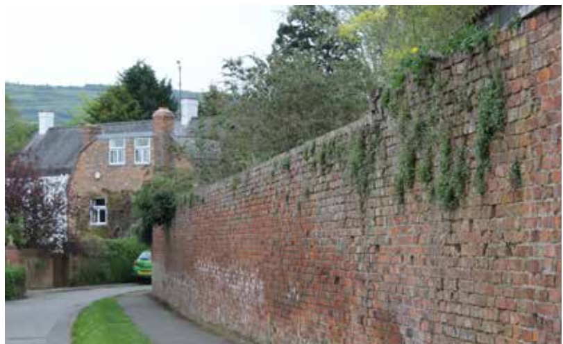
Fig.4.10 Brick Boundary Wall, Mill Street
