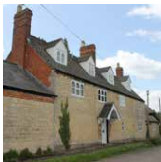
Fig.5.6 Lake House, Lake Street
