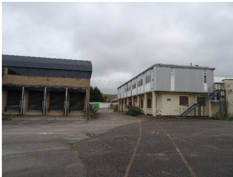
Photo 1: Example of buildings on Site.
