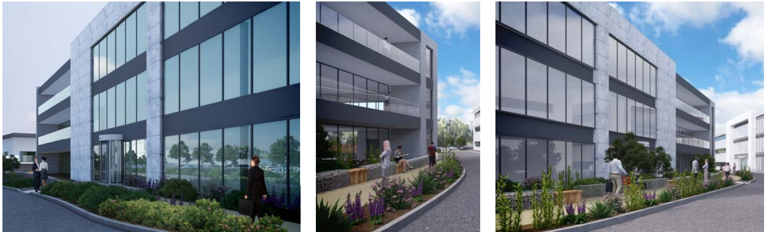
Views of Offices 1 and 2
