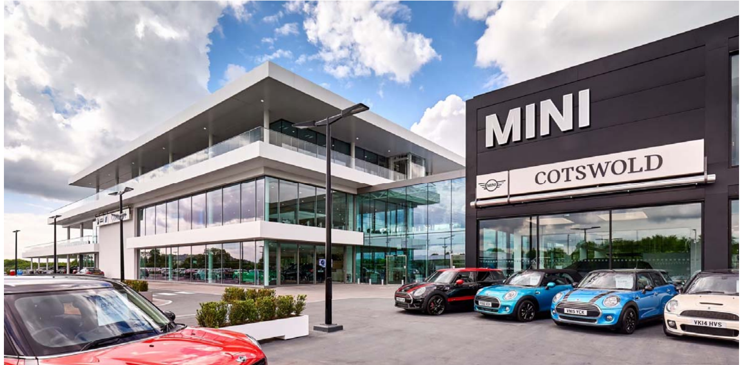
Recently completed BMW Mini Dealership
