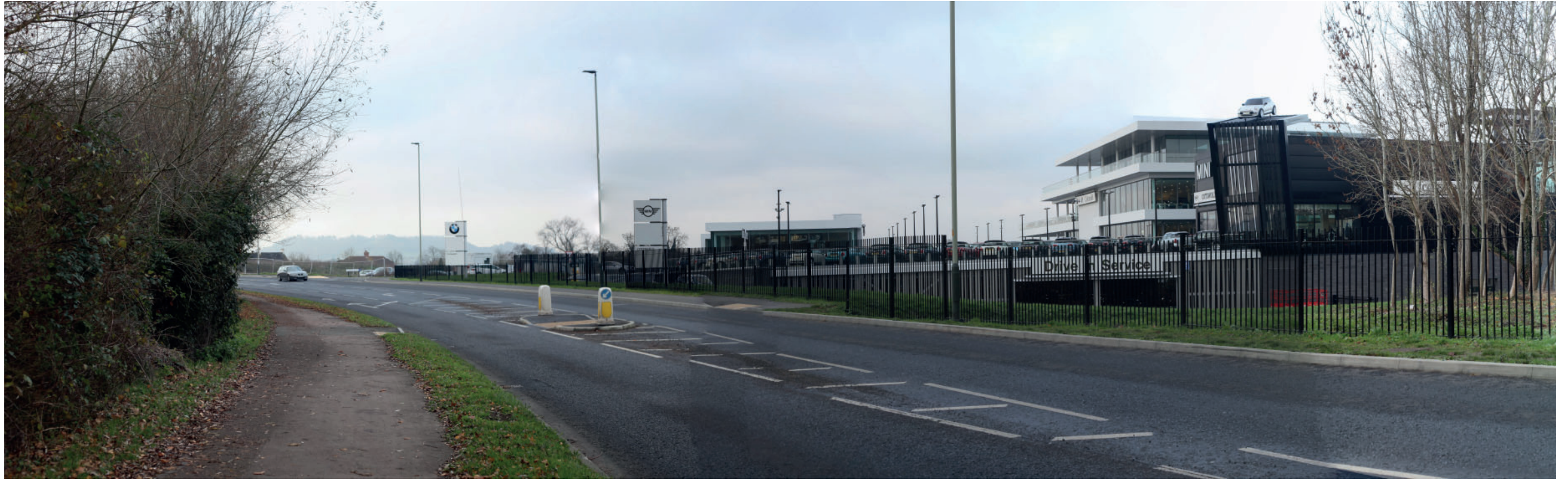
01: View towards site from approach on Grovefield Way to the northeast
