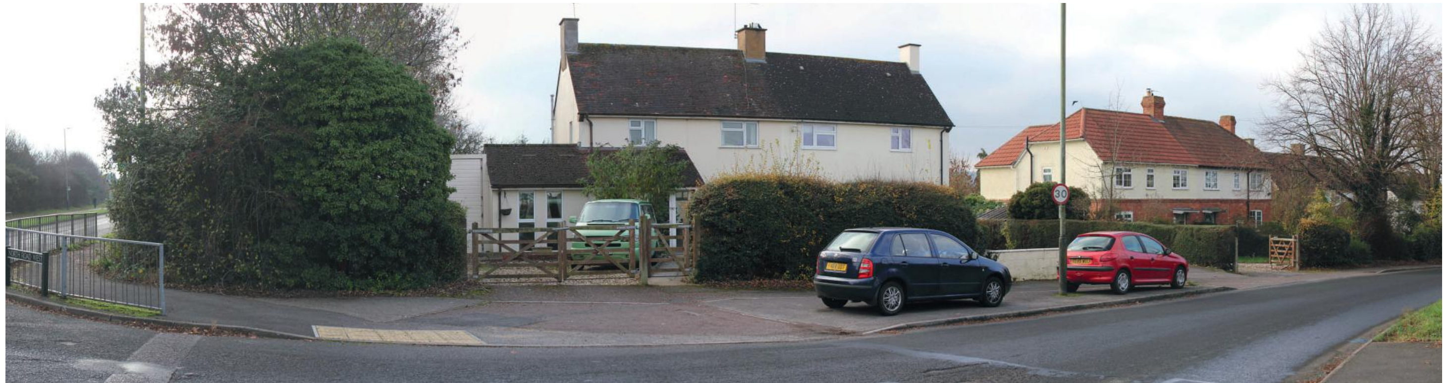
07: View south towards properties on North Road West
