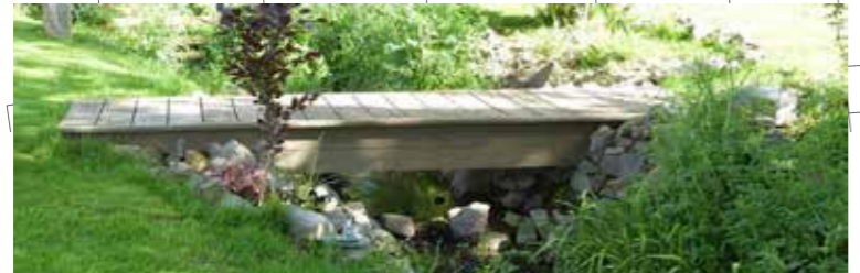
Indicative example of timber bridge off Kidnappers Lane over culvert 1.1m high timber guardrails required to tie into 1.5m high secure timber fencing to this location.
