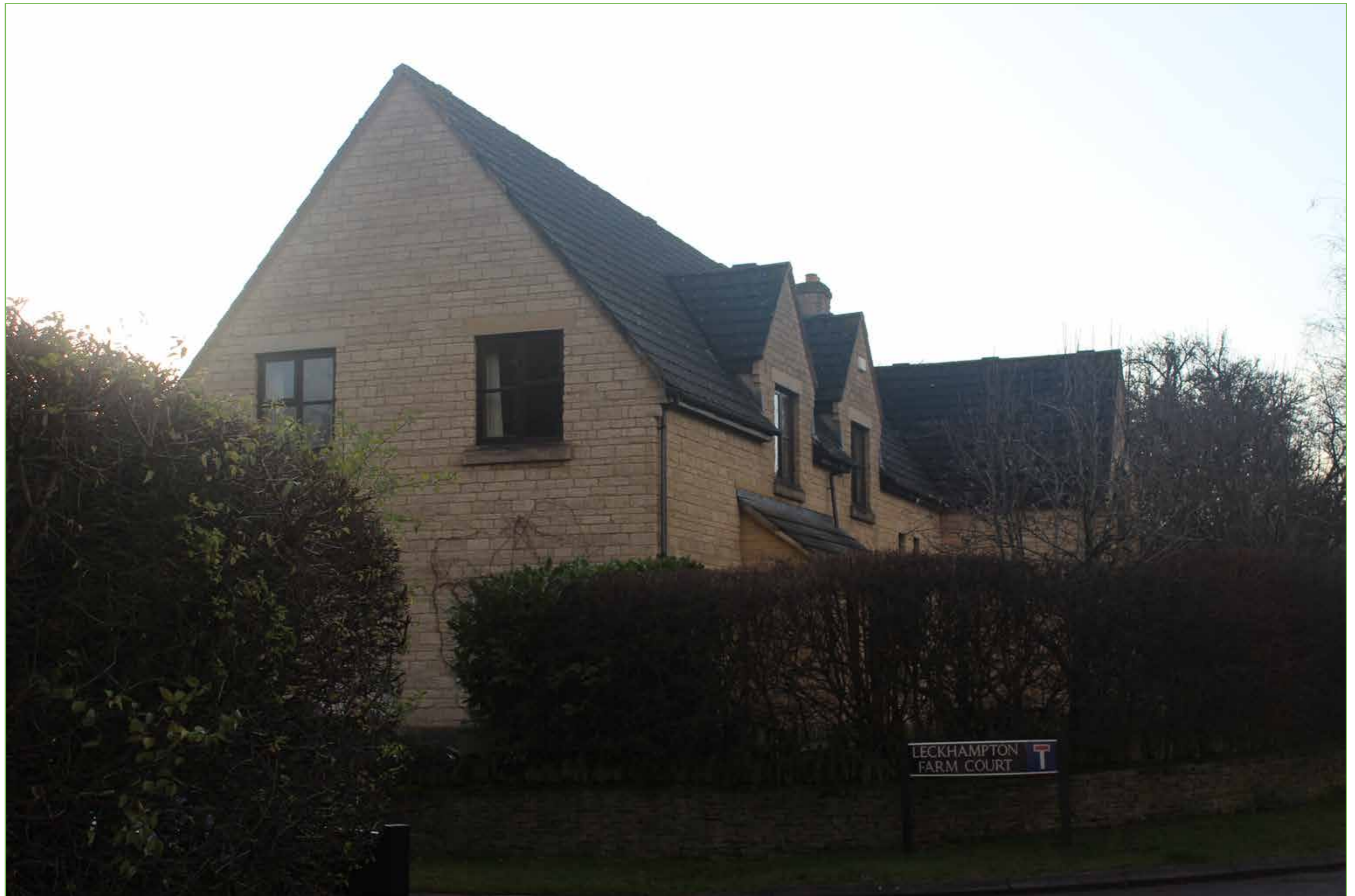
Appendix A: Figure 6 - Additional Photograph 4 View of new dwellings from Farm Lane at Leckhampton Farm Court 19186 Kidnappers Lane 25 Dwelling Scheme Appeal
