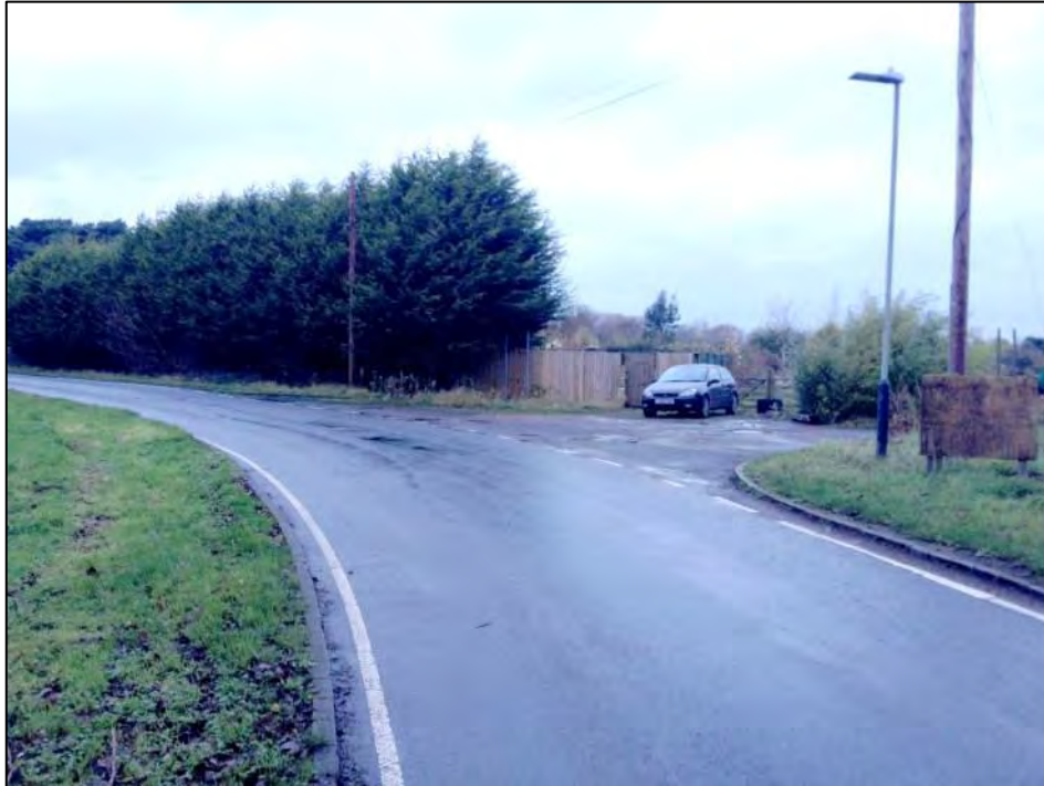
Photograph 3.1: Existing access to the application site
