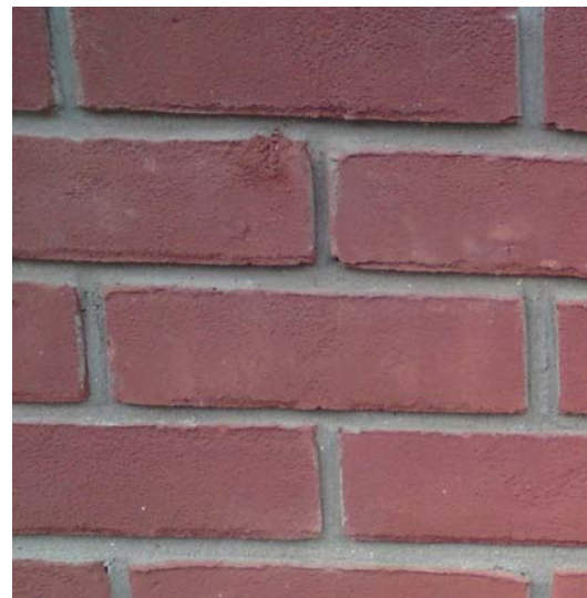
Figure 6. Good example of new facing brickwork. Showing slightly recessed pointing with the faces of the brick kept clean of mortar.
