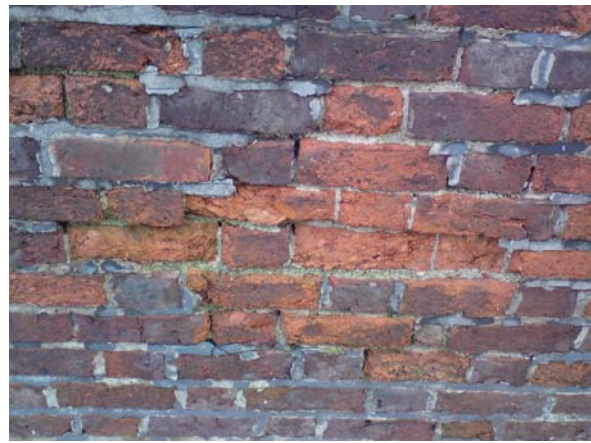
Figure 7. Bad example of pointing with cement mortar.
