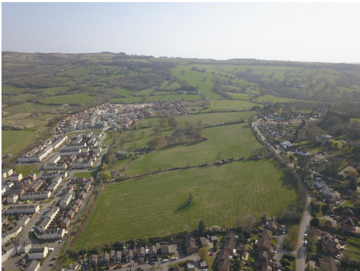
Fig 2. Hewletts Reservoir well-disguised.
