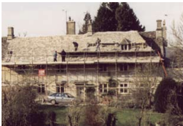
RE-ROOFING IN STONE SLATES
