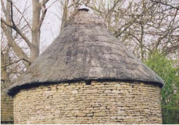
THATCH IN NEED OF MAINTENANCE
