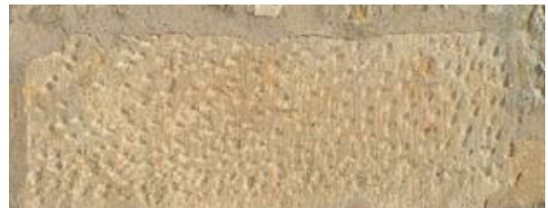
CHISELLED STONE WALLING
