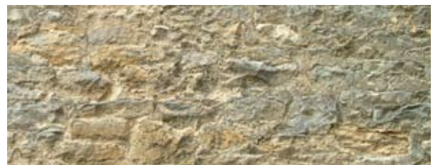
WALLING ('BUTTERED' STONE WALLING)
