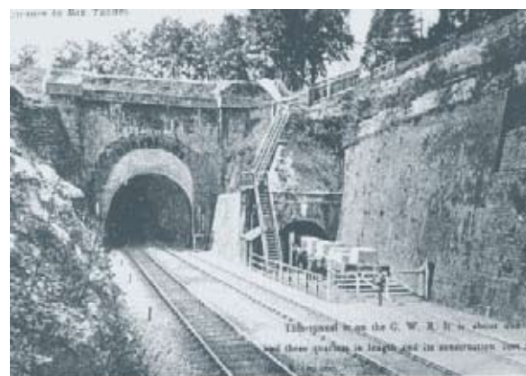
EAST PORTAL OF BOX TUNNEL SHOWING RAIL HEAD SERVING MINE
