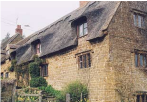
INAPPROPRIATE REED THATCH
