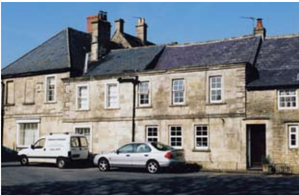
STONE SLATES REPLACED WITH WELSH SLATE
