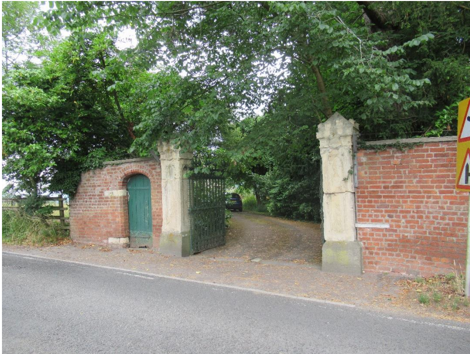
Fig.1 Entrance gates and boundary wall
