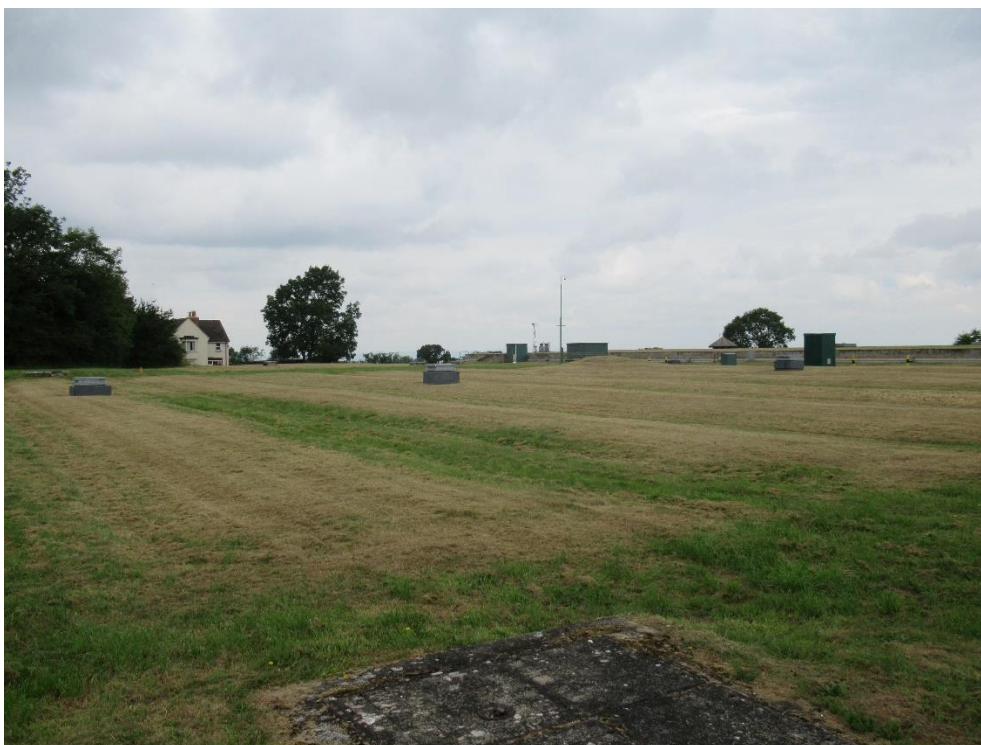
Fig.10 Covered roof over Reservoir No.2, looking west
