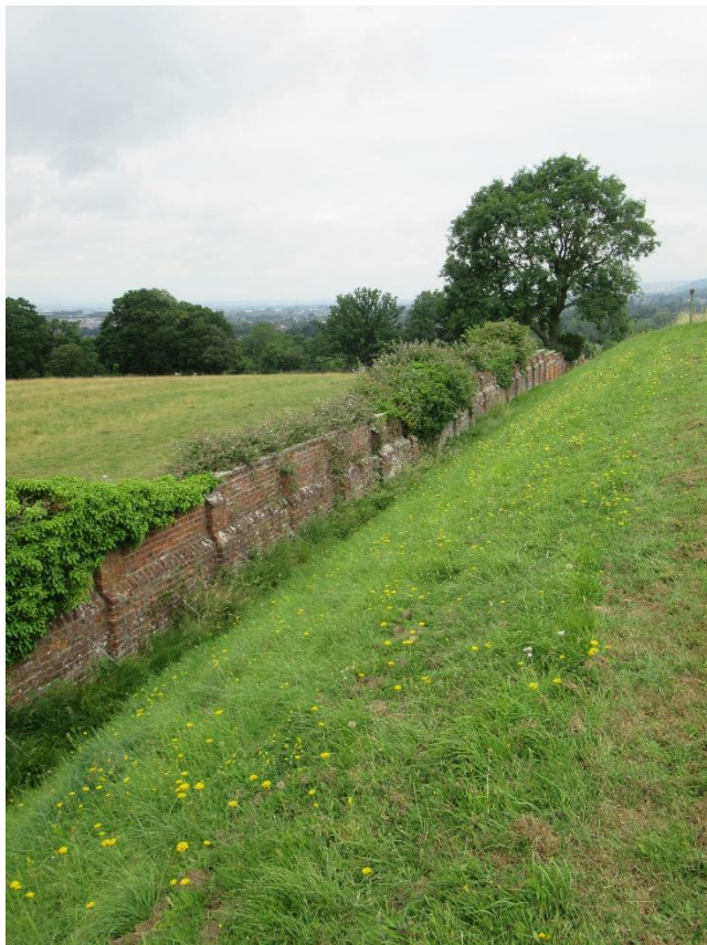
Fig.7 Buttressed brick wall and earth bank of Reservoir No.3.
