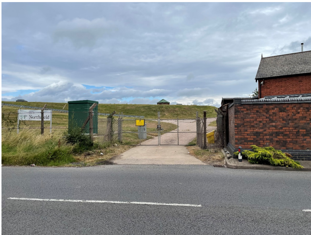
Figure 2 Photograph of structure at Northfield Reservoir – in exact position of valve house shown on mapping above
