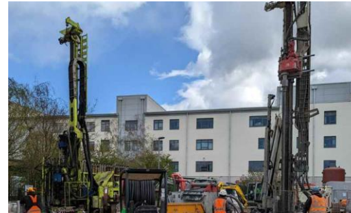
Gloucestershire College, Ground Source Heat Pump borehole drilling
