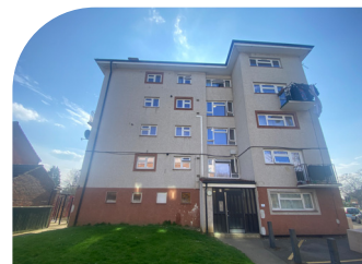
Before and after images of the flats at Arle Road, Grevil Road and Orchard Way.
