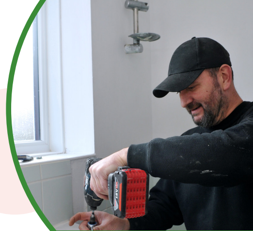
Louis Fletcher, multi-skill operative, repairing a bathroom tap.
