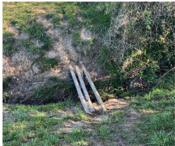
Photo of informal footbridge over brook inhibiting accessibility
